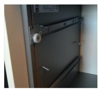
Fixate the Set of drawers in the cabinet or the tower through the pre-drilled holes in one of the sides of the drawer set. Use the two screws in the plastic bag that lays in one of the drawers.
